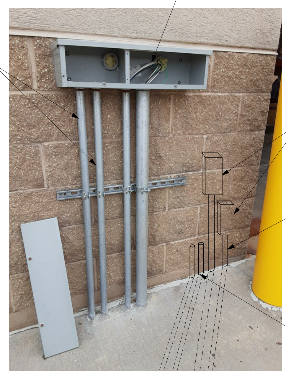
4 Exterior Junction Box/wiring NTS
